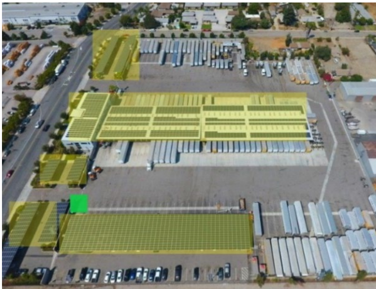
Figure 22: Solar Panels Installed at DHE
