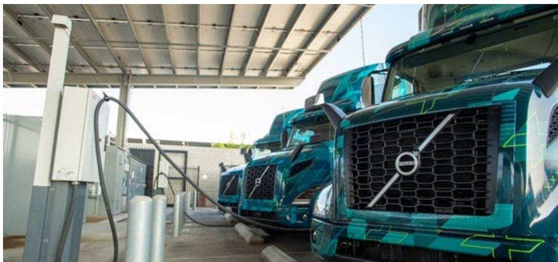
Figure 18: Class 8 Tractors at DHE Facility
